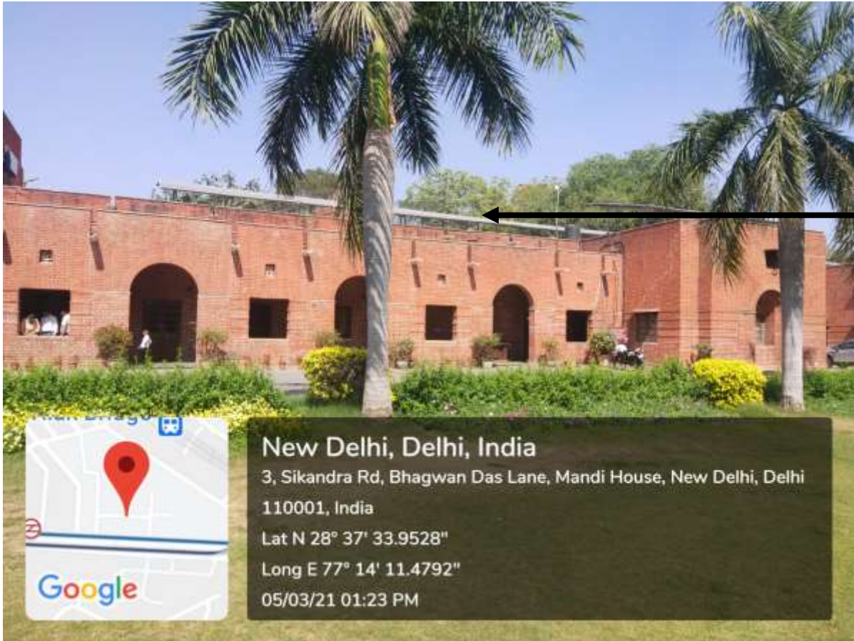
SPV Panels on college rooftops
